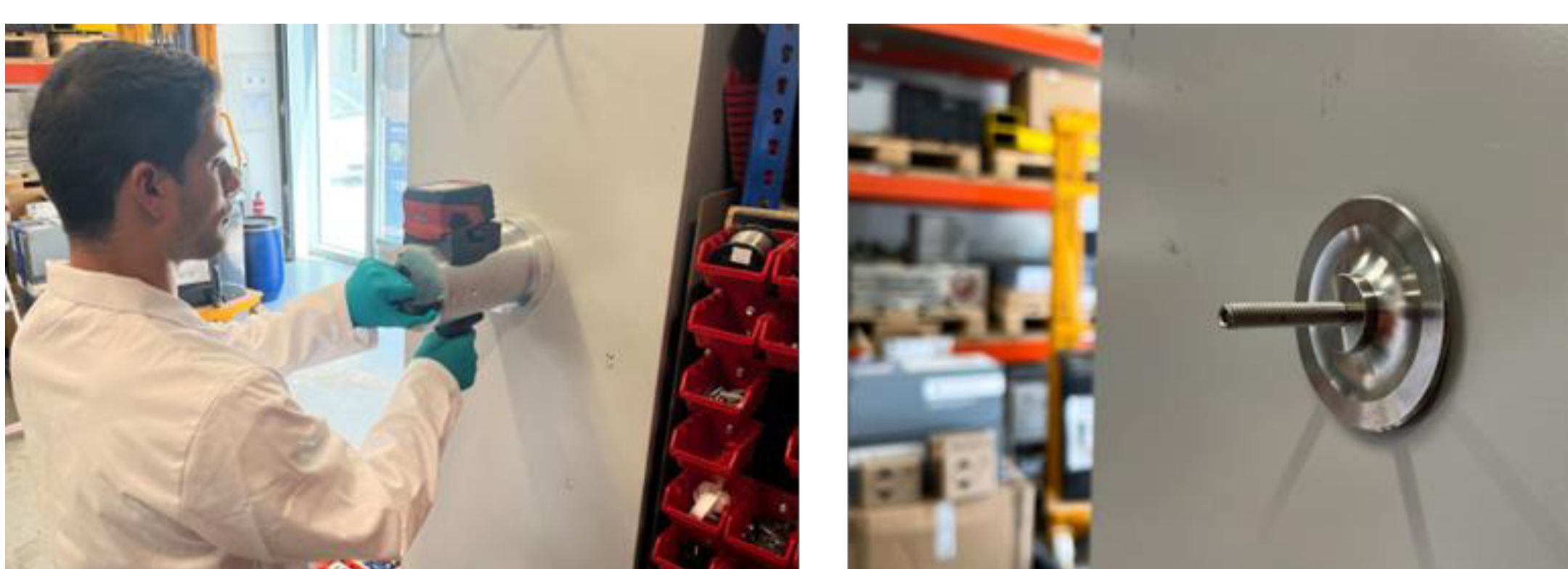
Installation of a fastener with the automated tool
