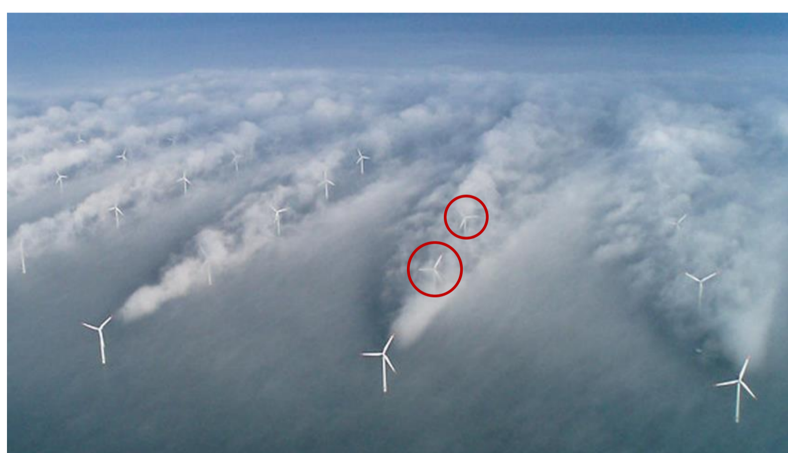
Horns rev 1 (DK) offshore wind farm (160 MW – 80 V80 – 2.0 MW) © Christian Steiness, Vattenfall – 2008
